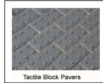
Concrete pavers for footways and cycle ways can be 50 mm thick, for places where motor transport will cross the pavers a minimum of 75 mm thickness is needed,
